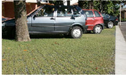
Figure 10. Open mesh porous paving supporting vegetative cover
