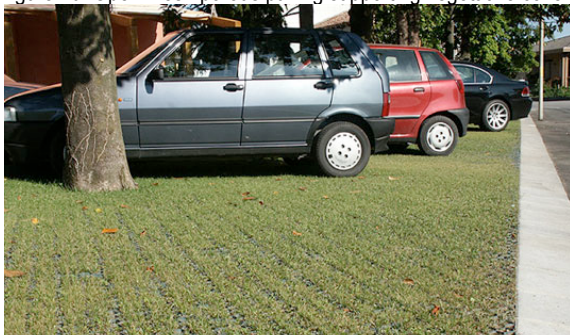
Figure 10. Open mesh porous paving supporting vegetative cover
