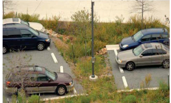
Figure P5. Use of vegetation strips in parking lots collects and filters runoff, but also provides a more attractive and cooler parking surface.
