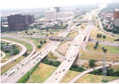
Dallas freeway interchange
