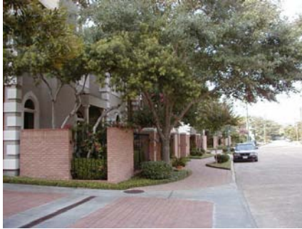
Pervious brick pavers on sidewalks and driveways
