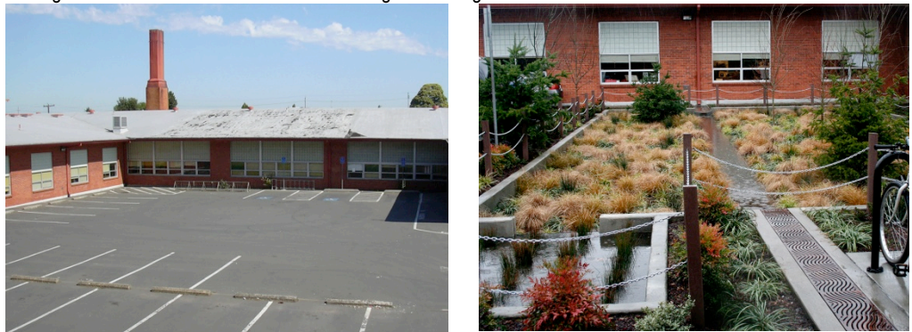
Figure P8. Previously paved street segment converted to water infiltration planter; Portland Raingarden and Ecosroofs Programs. 98
