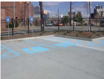
Porous paving parking lot
