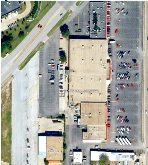
Figure 3. Dallas commercial site
