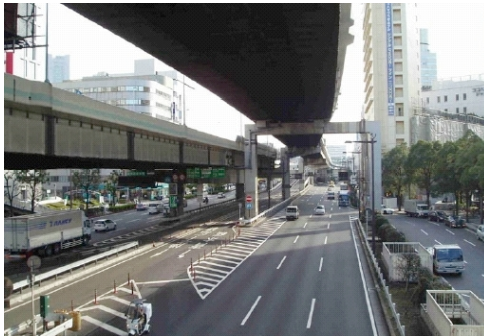
Porous paving highway in Japan
