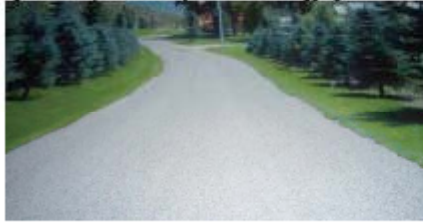
Figure 11. Chip Seal Overlay with Reflective Aggregate
