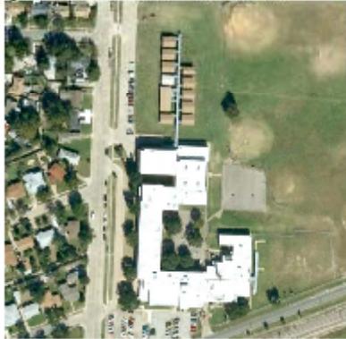
Figure 9. Dallas School with Cool Reflective Roof
